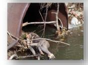
Culverts are also critical drainage structures that carry the natural flow of water under the road so that the water can continue on its natural course and should be kept free of debris, silt and eroded soil. Cleaning of the outlet of culverts to ensure free-flow conditions on the downstream side should also not be neglected.
