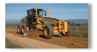
Spot re-gravelling can also be carried out to replace the gravel over localised areas where it has become excessively thin and for the filling of potholes, ruts and erosion channels. This is another function that can be effectively used to increase the labour component as part of the maintenance program.
