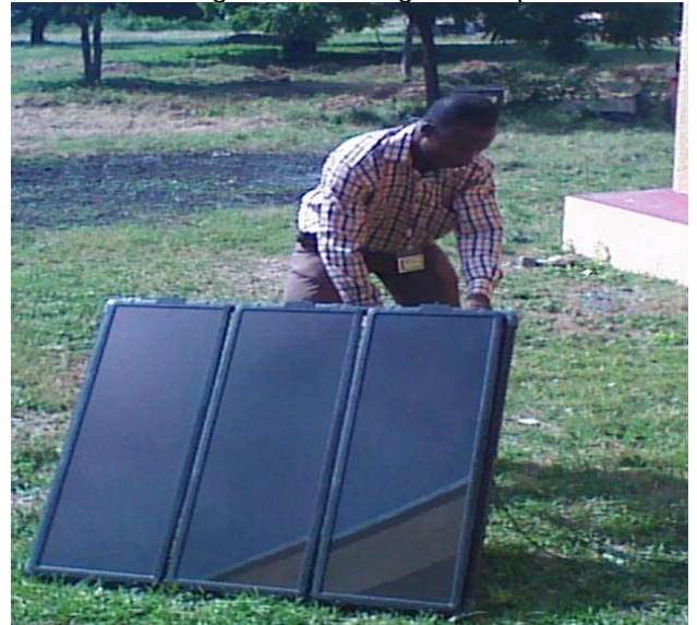
KERSL engineer installing a solar panel
