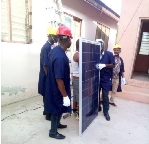
Training in solar power installation
